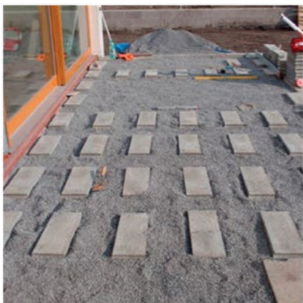
compacted gravel bed
